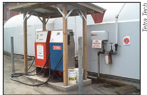
Figure 8. Spill kits should be maintained in areas with spill potential, such as fueling stations.
